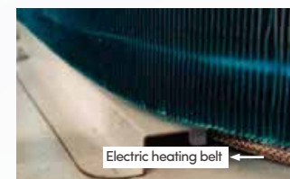
Third design: Water and electricity heating belt in heat exchange chassis
